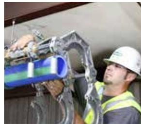
**LIGHTWEIGHT** Initially weighing just 40 pounds in the 4-jaw configuration, the Acrobat lightens the load to a mere 29 pounds in its 3-jaw configuration – making overhead fusions a breeze.
